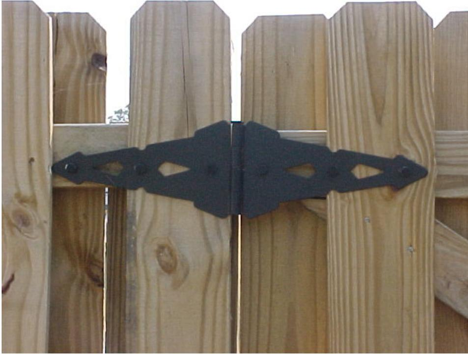
Photograph #5: Standard Gate Hinge Hardware
