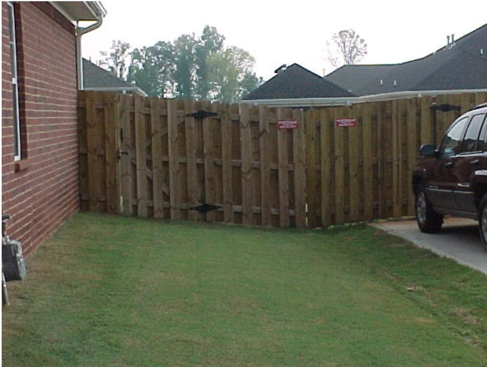
Photograph #4: Standard Fence Fitted to Property Slope
